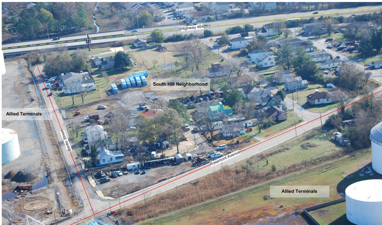
Photo courtesy of City of Chesapeake Fire Marshal
