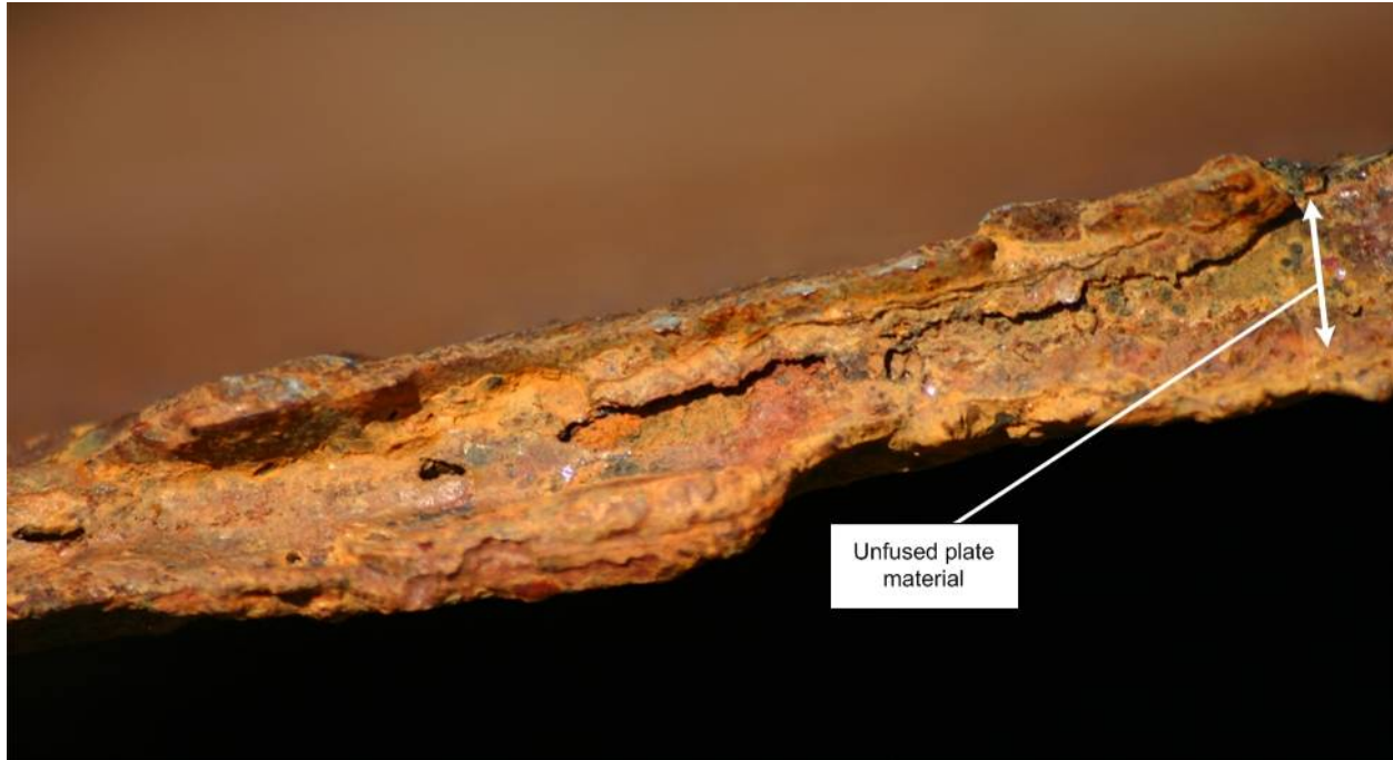
Figure 10. Failed tank weld on course three.
