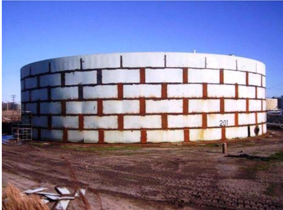
Photo from HMT inspection report.
